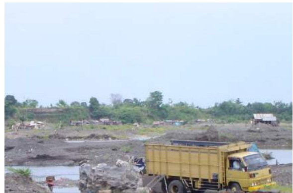
Figure 1. the sand excavation of Gunaksa Bali.
