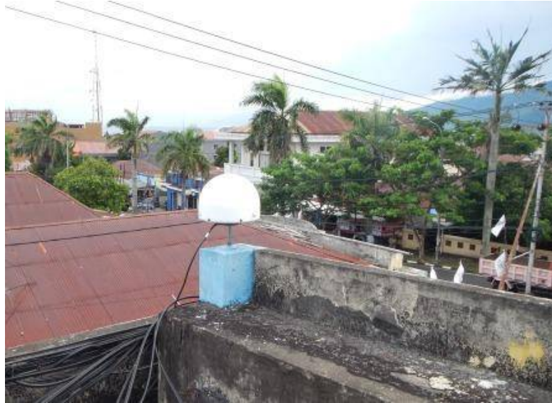
Gb-13. Antena Base Station CTER Kota Ternate.
